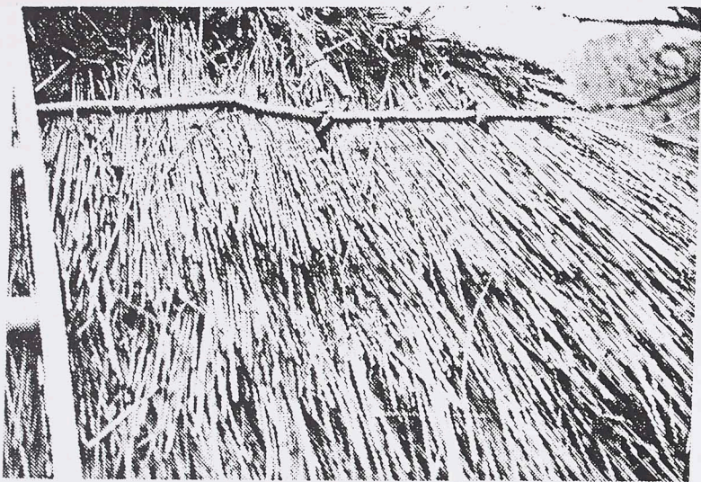
Lath and pegs securing course of thatch
