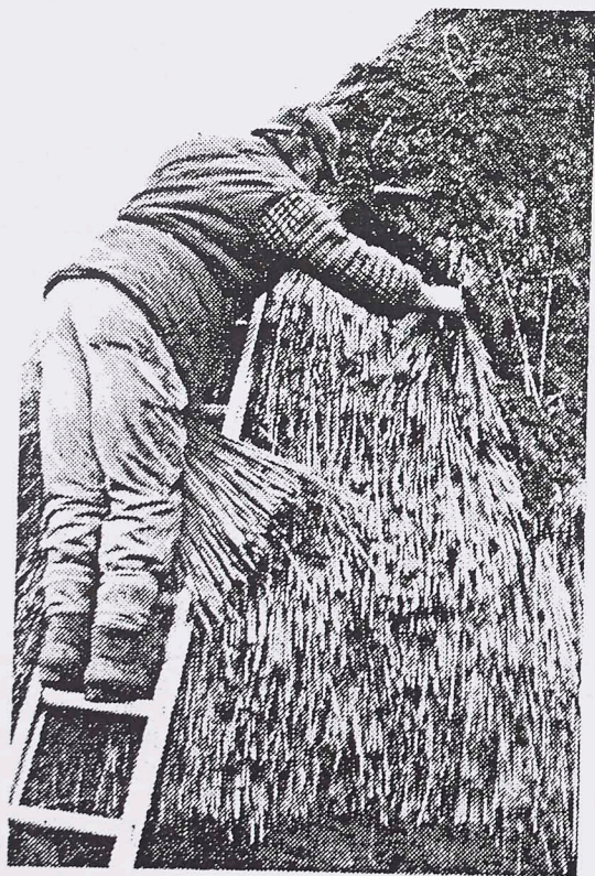
Lath and pegs securing course of thatch
