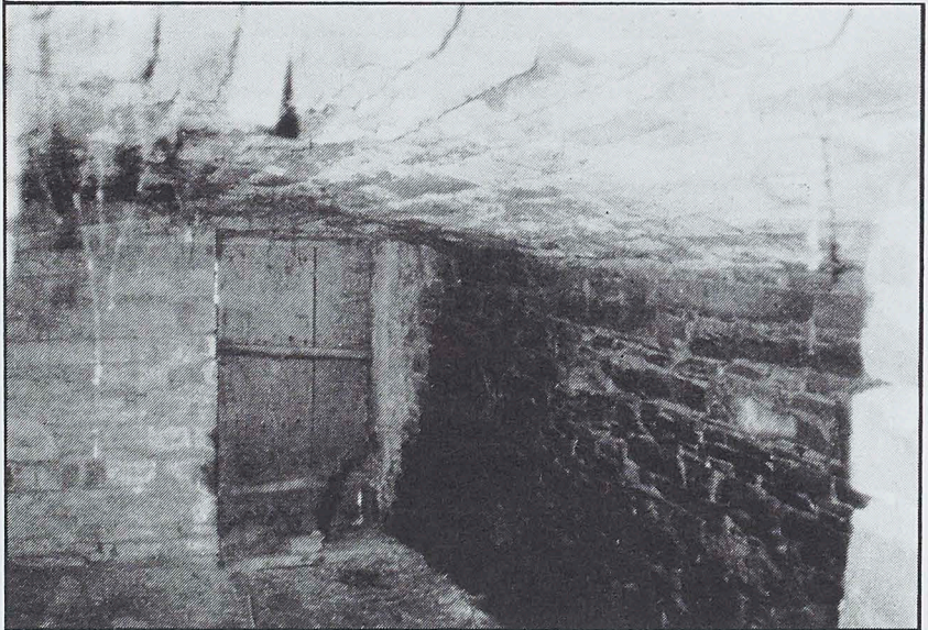
The threshing barn, showing the segmental vaulted chamber with battered walls
