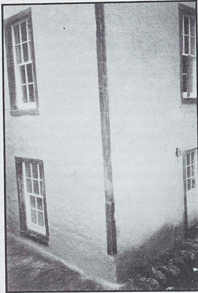
West and South Elevation : Completed Harl The West elevation finished with lime wash
