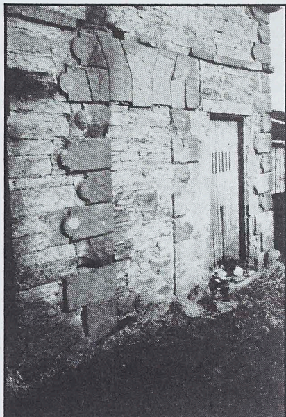
Buckle-type quoins in the former threshing barn
