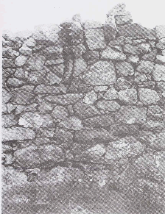
figure 8 Croft house at Glendrian, south gable with remnant of end cruck and protruding stones to
