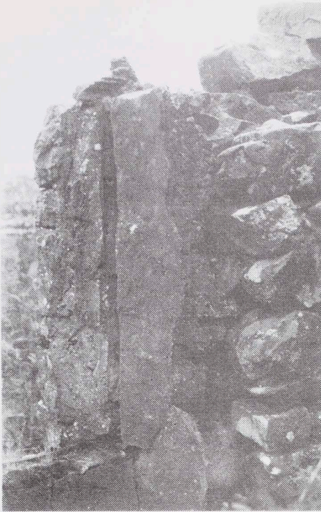
figure 3 House at Camas nan Geall, cruck slot adjoining window opening
