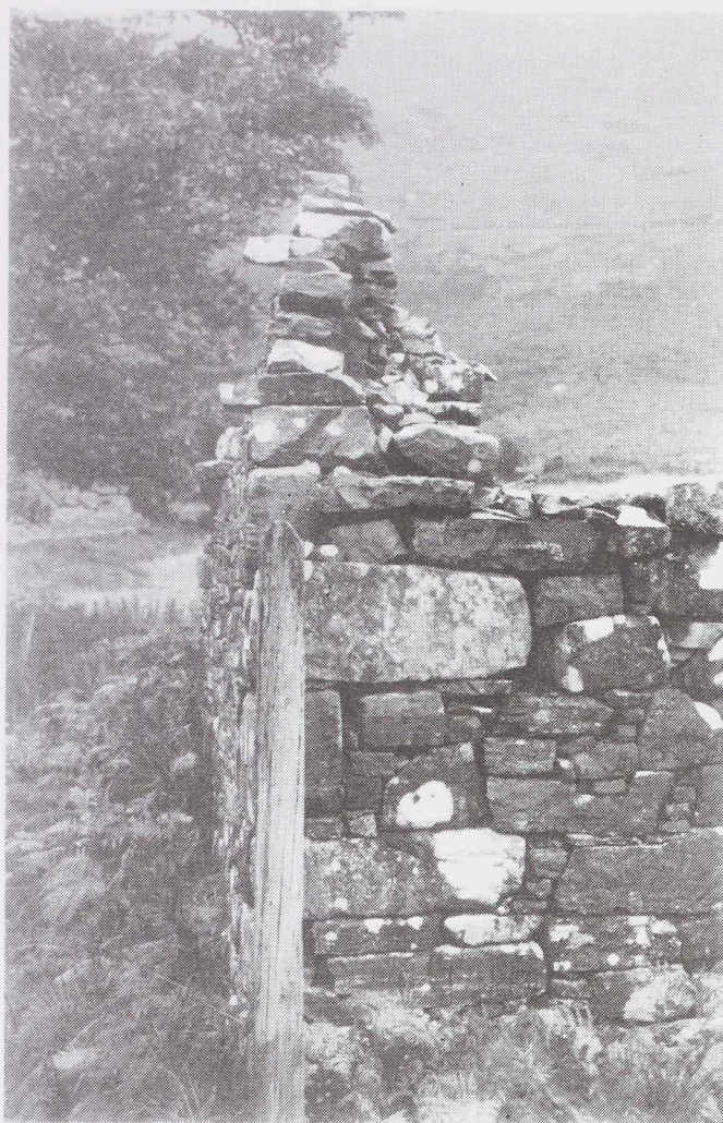
figure 4 House at Camas nan Geall, west gable with stone thatch
