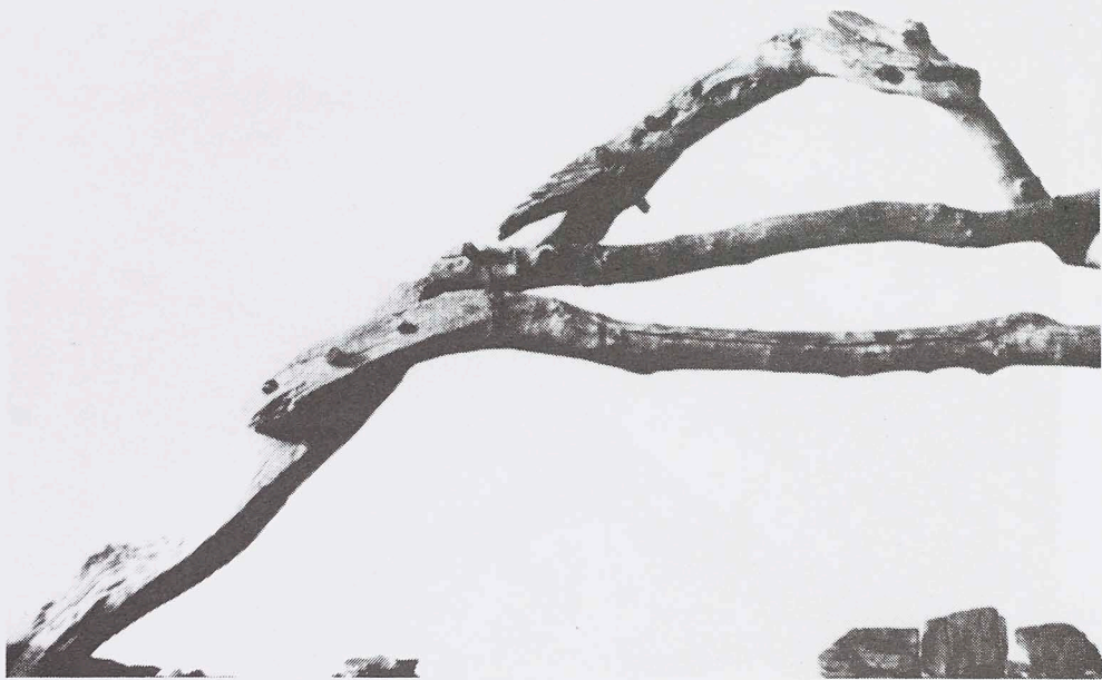
figure 3 Slettil, a house in an advanced state of decay, last standing couple
