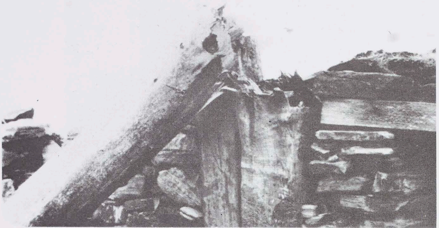
figure 6 Slettil house, cruck frame smashed by gale, and timber window lintel
