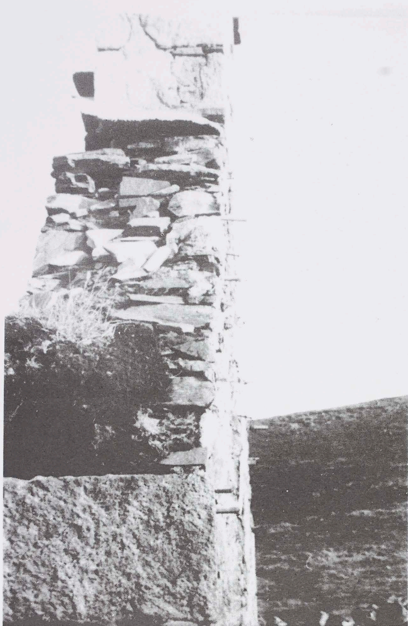
figure 8 Slettil house, showing thatching pegs set into gable to secure horizontal ropes
