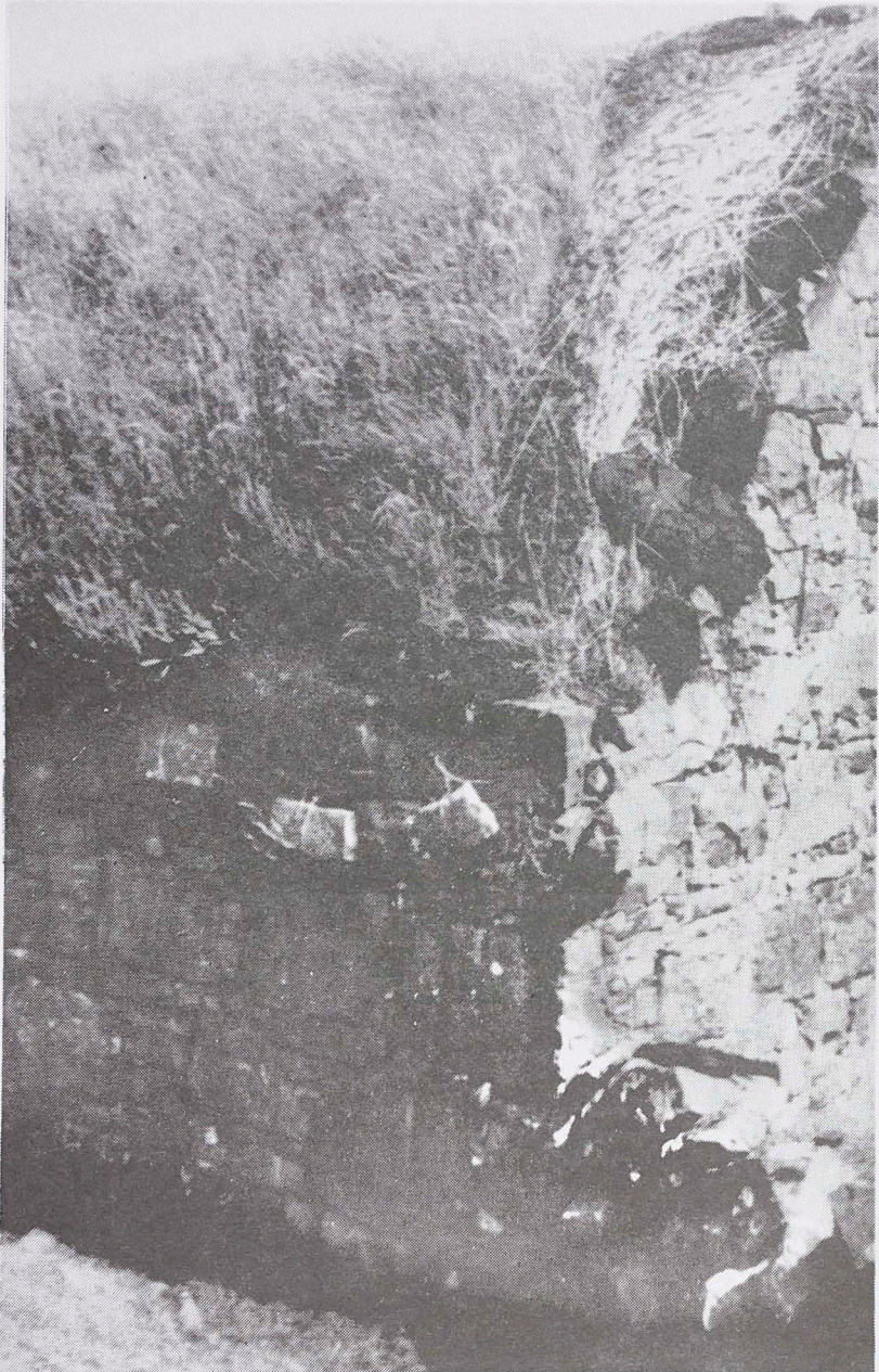
figure 7 Stoer house, showing weighted ropes across roof and thatching pegs
