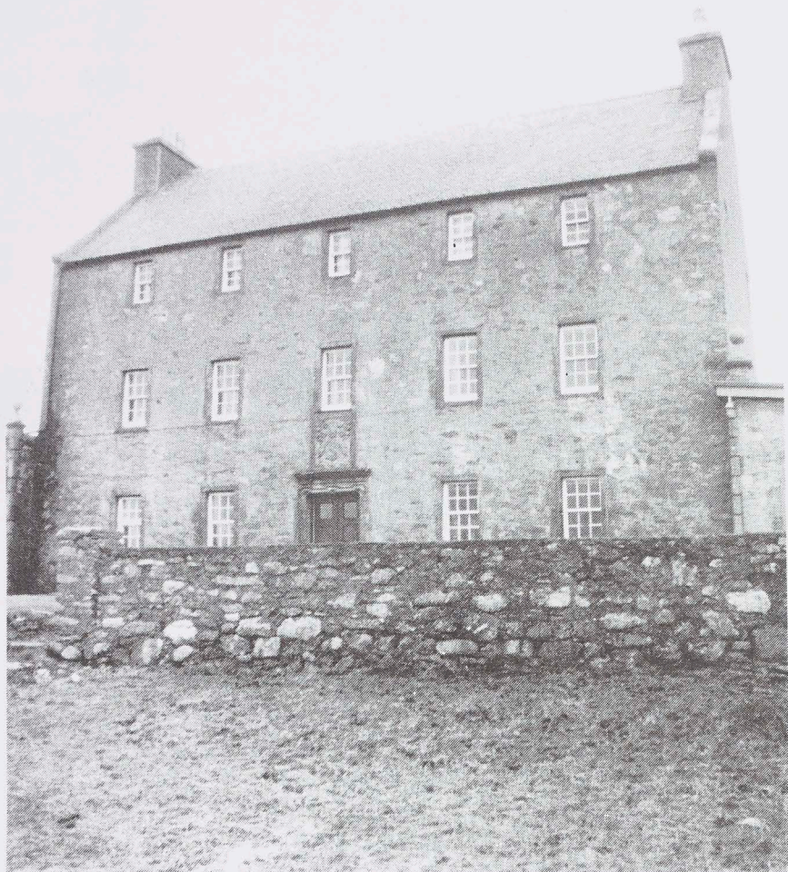
figure 7 The Haa of Sand, West Mainland. Perhaps the ultimate development of the Shetland Haa, dating from 1754. A tall three storey, five bay wide Haa. The entrance door has a shouldered architrave with an armorial panel above it. Symmetrical single storey wings at either side of the Haa (now altered) each have a ball capped apex. The principal rooms on the first floor are indicated by their large windows; smaller windows serve the second floor bedrooms. All first and second floor rooms retain their fielded panelling with arcaded panelling in the drawing room. Almost unaltered internally other than the ground floor where the staircase has been turned and the entrance hall enlarged. The Haa was built as a summerhouse by Sir Andrew Mitchell of Westshore (Scalloway) who was given leave by the Earl of Morton to remove from Scalloway Castle 'dressed freestones torn from their place to supply door and window jambs and lintels, and cornerstones for this mansion' 3 . Two complete doorways from the castle lead into the walled policies.
