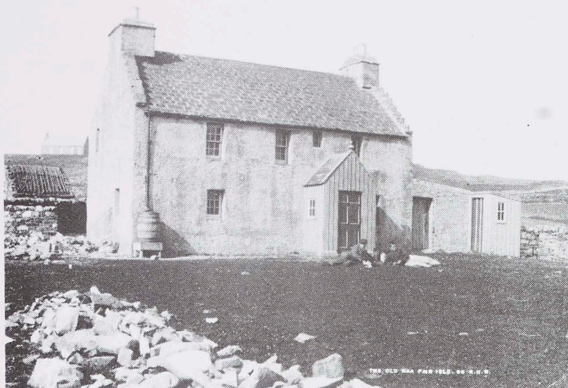
figure 3 The Haa, Fair Isle. Eighteenth century. A small solid looking Haa with windows placed irregularly on the front elevation. The gables are crow-stepped, and the roof timbers are said to be from wrecks. The Haa was built as the factor's house by the Stewarts of Brough (Orkney), who acquired Fair Isle in 1766. A fine early Haa, probably more influenced by Orkney building traditions than by those of Shetland. (Photograph - Shetland Museum)
