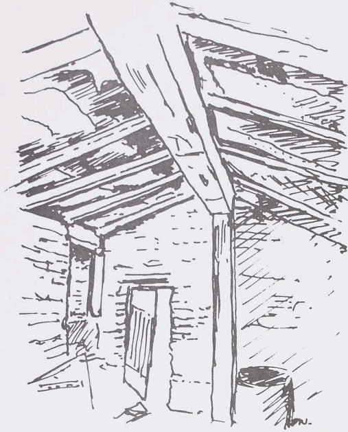
figure 7 Interior of Verracott barn showing maintree and kiln opening on left
