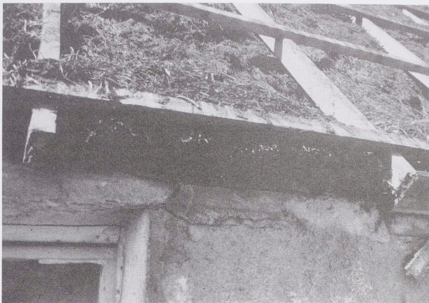
Figure 4 Detail of thatch at eaves
