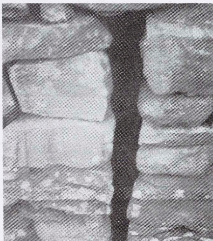
Figure 6 Cattybraes: (a) gable wall showing slit; detail (b) inside, covered with flag held by metal clips, (c) outside, with clay clearly visible.
