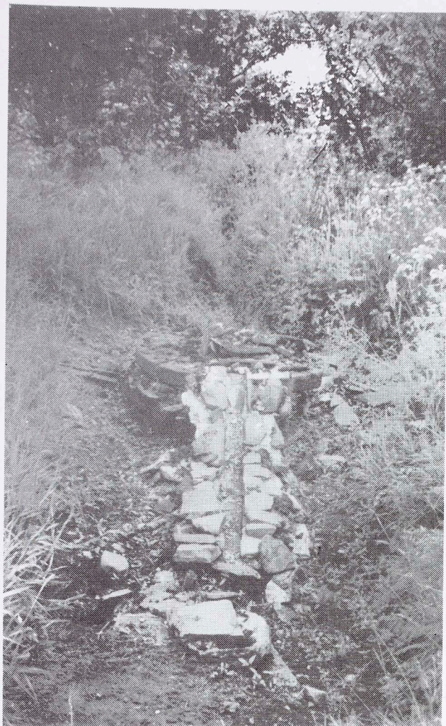
Figure 5 Second cupola site base; note chute for pouring molten cast iron.
