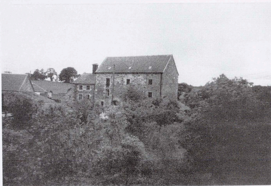
Figure 2 The mill building comprises (left to right) lean-to kiln fuel store, later converted to farm dairy; grain-drying kiln; main mill with domestic dwelling incorporated in left-hand side and fully workable mill machinery retained to the right; lean-to waterwheel house. The main road used to pass between the mill and the farm buildings on the left.
