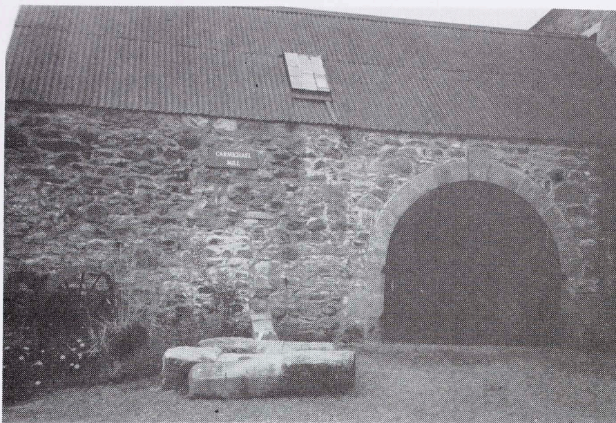
Figure 6 Possibly the earliest building on the site. Perhaps once a two-storey farm building, then converted to a bothy for the mill workers, it had a doorway in the gable end adjacent to the mill and a stairway leading to the back door of the mill. Later still, the first floor was removed and the ground floor raised, possibly because of flooding (as was the main mill floor), and it became a cattle byre and cart shed. The corrugated metal roof sheeting and roof pitch could indicate its being originally thatched
