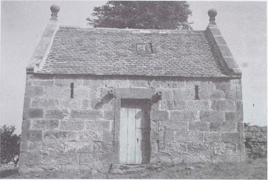
Figure 3 The slaughter house, Craigston; harling was only used on the rubble walling, not on the front.
