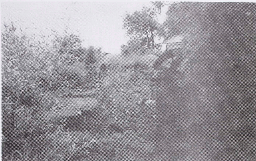
Figure 3 Pre-improvement grain mill c. 1720, originally with an external waterwheel on the gable wall nearest the river. It would have had a single set of millstones and primitive gearing. It later became a lint mill (c. 1760–90), with a wheel mounted internally, then the site of an iron foundry (c. 1790).
