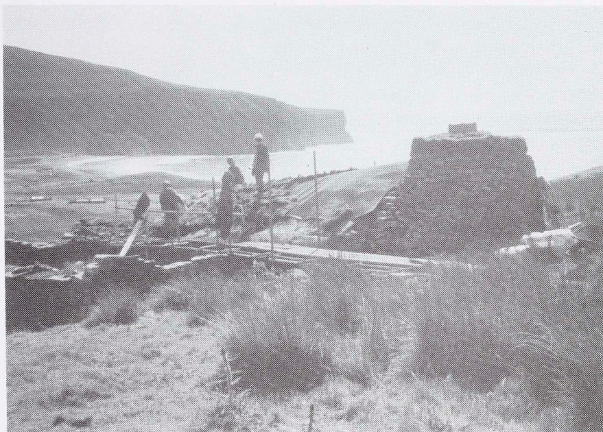
Figure 4 Reconstruction in progress: turf being placed over the geotextile membrane.
