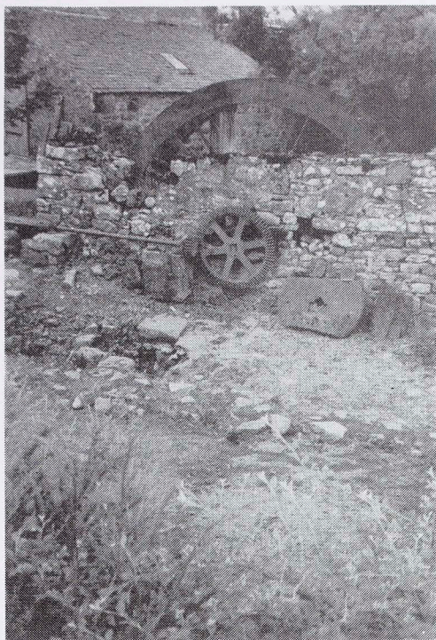
Figure 4 The remains of the foundry site, showing the drive shaft from the waterwheel repositioned at 90 degrees to transmit power to drive a farm threshing mill. It originally passed straight out from the centre of the waterwheel to drive foundry machinery including bellows, tilt hammers and grindstones for edge tool production. Centre left is the foundation of a cupola, with slag heap behind and casting floor to the front; the broken kibbling stone leaning against the wall was used as the cupola base.
