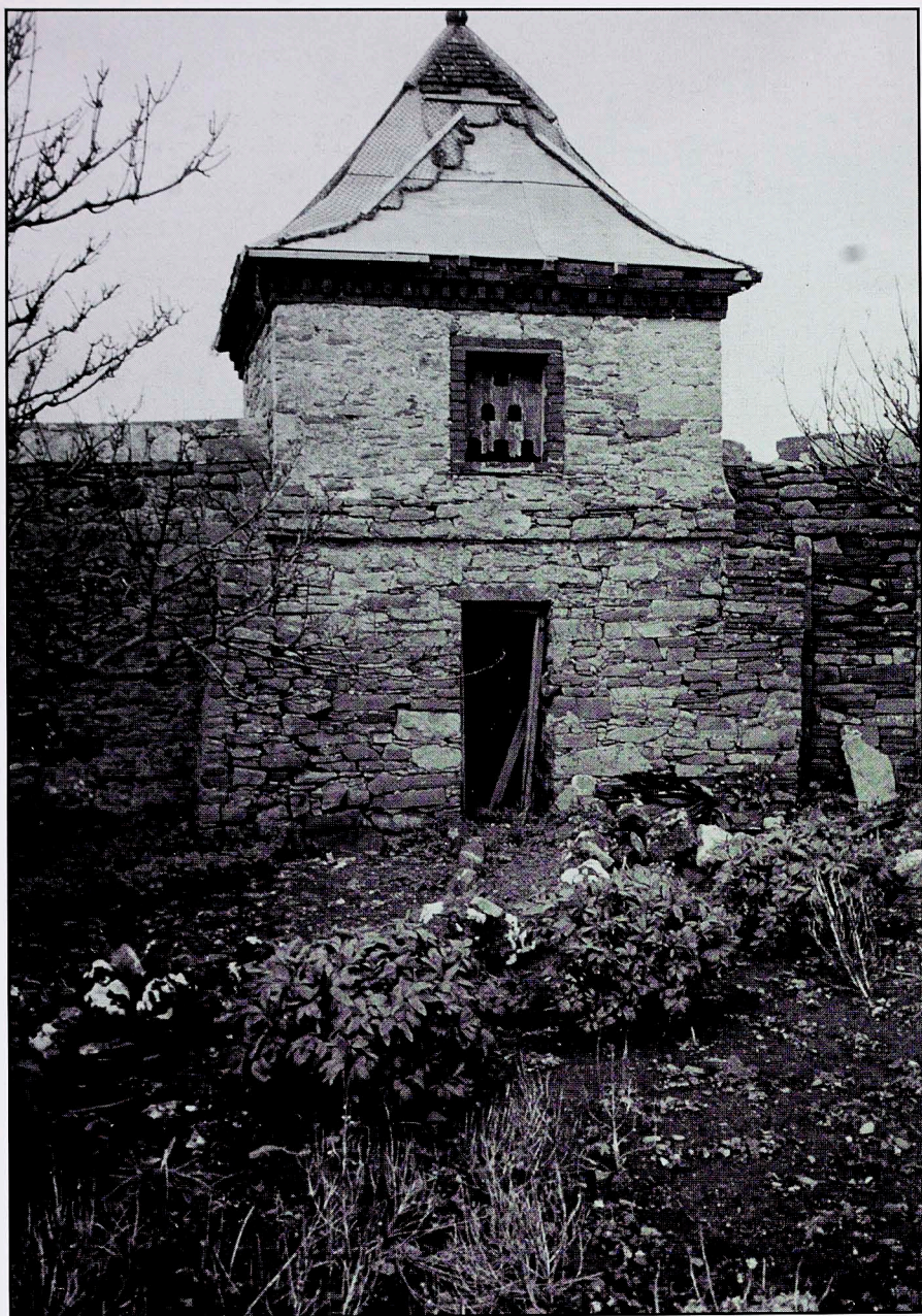
Figure 4 South elevation, showing the narrow but tall central ground-floor door for human access, with the brick-edged aperture containing timber flight-holes for pigeons above. Although the structure is rapidly deteriorating, much of the harling finish on the upper chamber wall is still visible between the dentilled brickwork eaves and the stone bandcourse.
