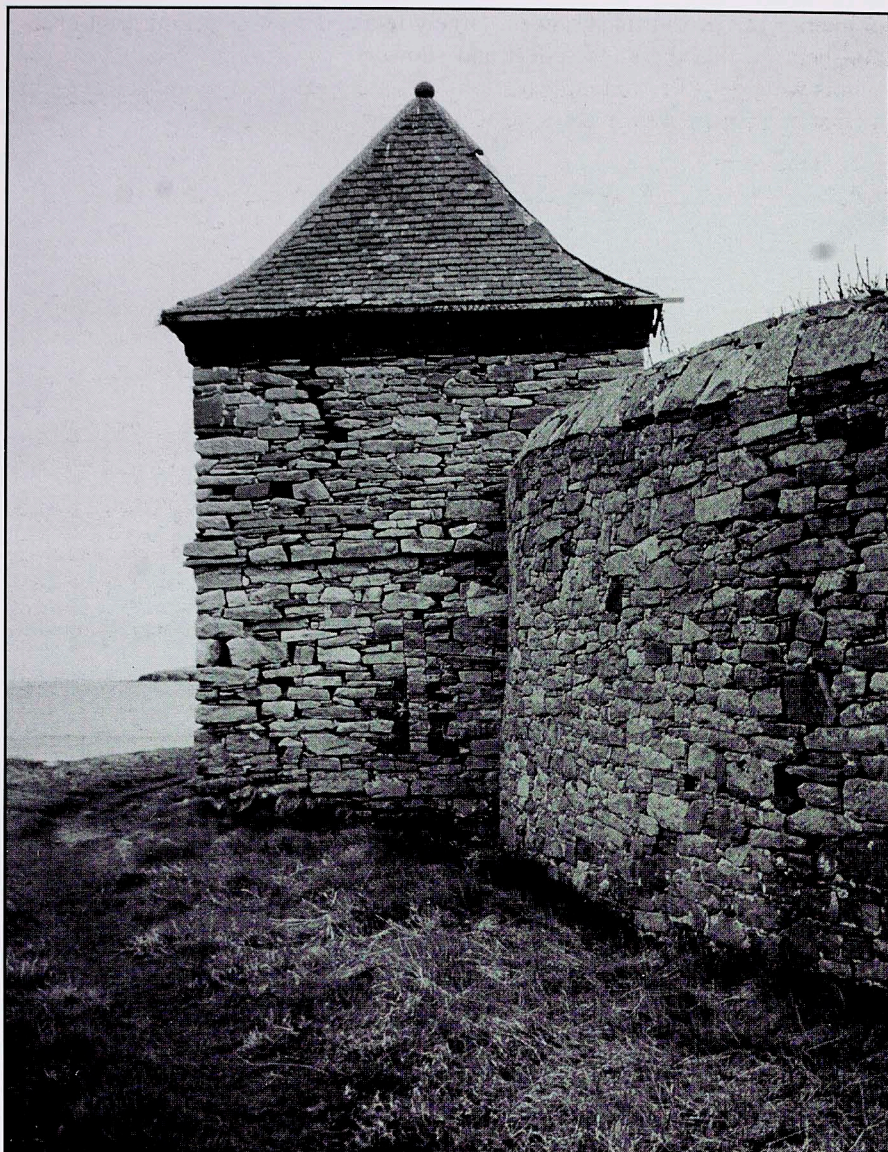
Figure 5 View from the west, showing the relationship between the doocot and the later garden wall. The sweep of the pavilion roof is very evident, but the blocked slit window on the ground floor is barely visible. Sadly, cracks in both the doocot and garden walls are beginning to develop.
