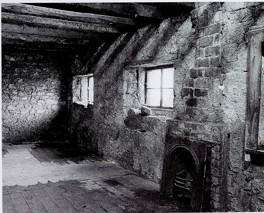
Figure 12 Interior of No. 11, showing back (east)-facing windows before loose material and stonework was removed from the sills.
