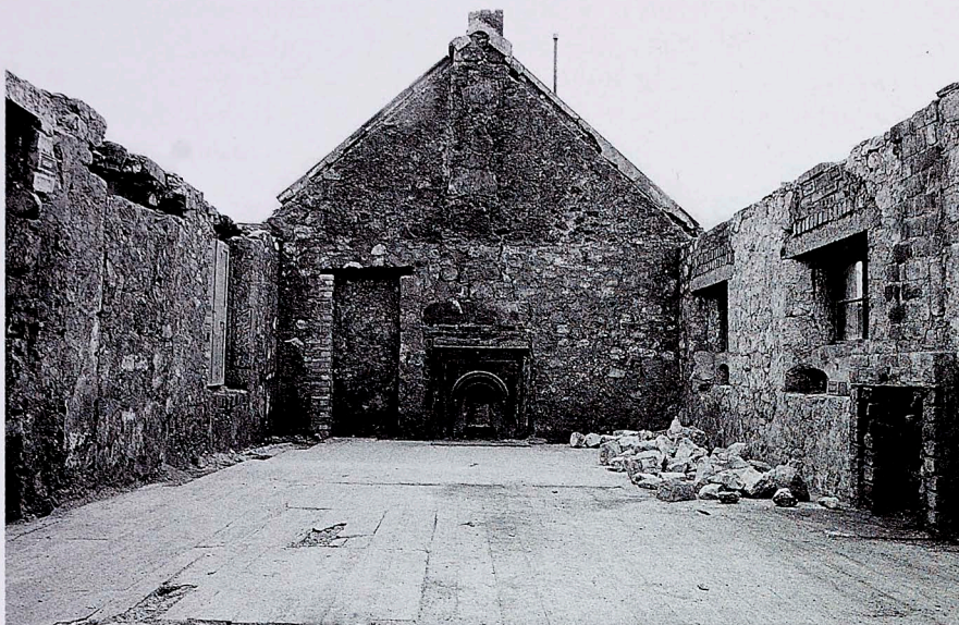
Figure 14 Interior of No. 11, looking toward north gable, showing rough masonry and a blocked up window in the western wall (left).
