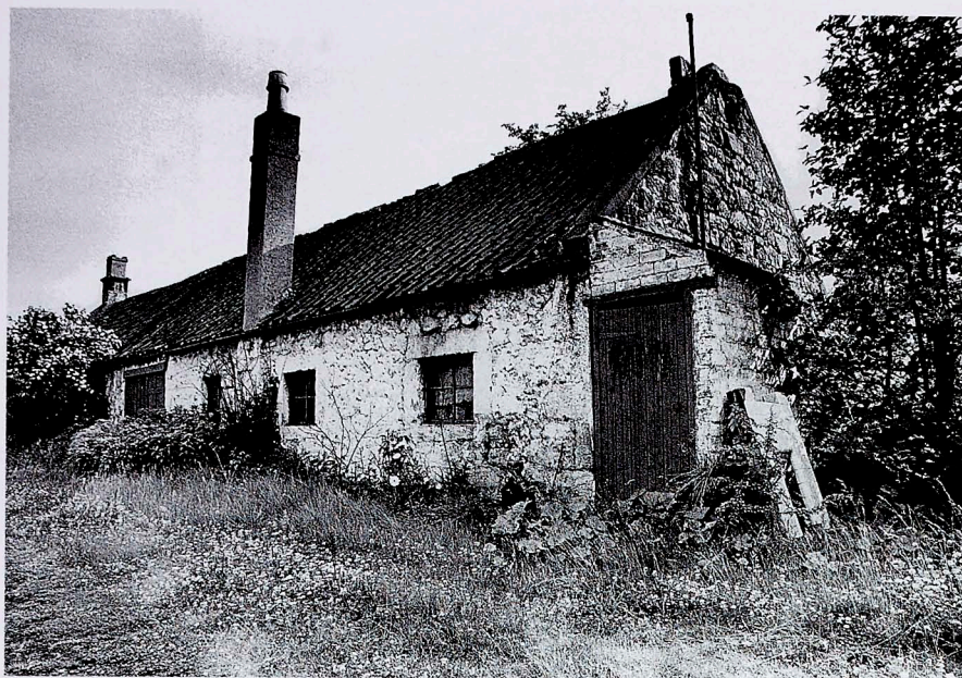
Figure 18 Closet attached to north gable; this gable contains a high proportion of field boulders.
