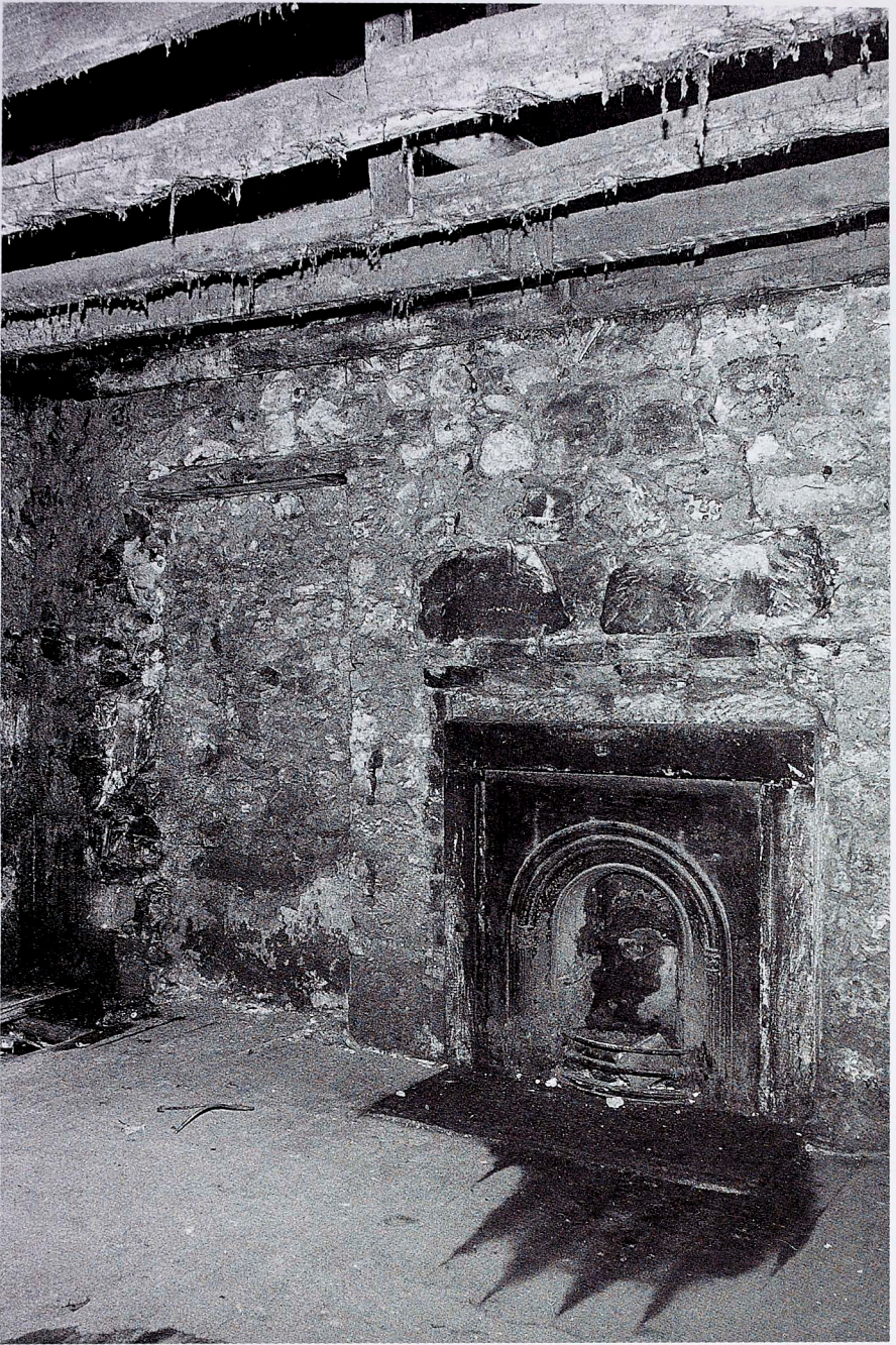
Figure 11 Interior of No. 11, showing north gable fireplace; note the larger space filled-in with bricks and the keystone arrangement above the Victorian fireplace lintel.
