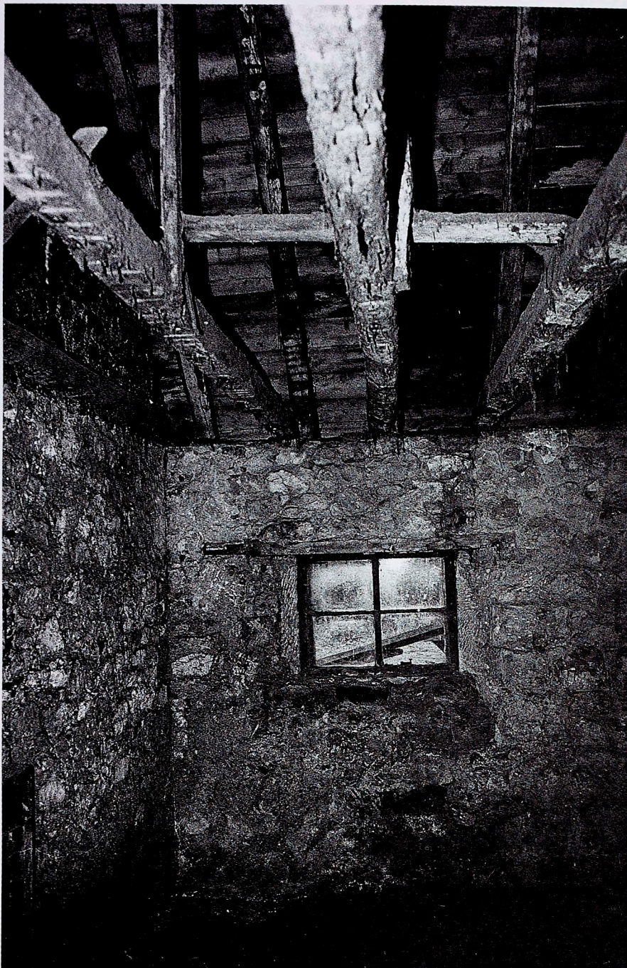
Figure 3 Interior of No. 11, showing the tree beams near the northeast corner of the north gable.
