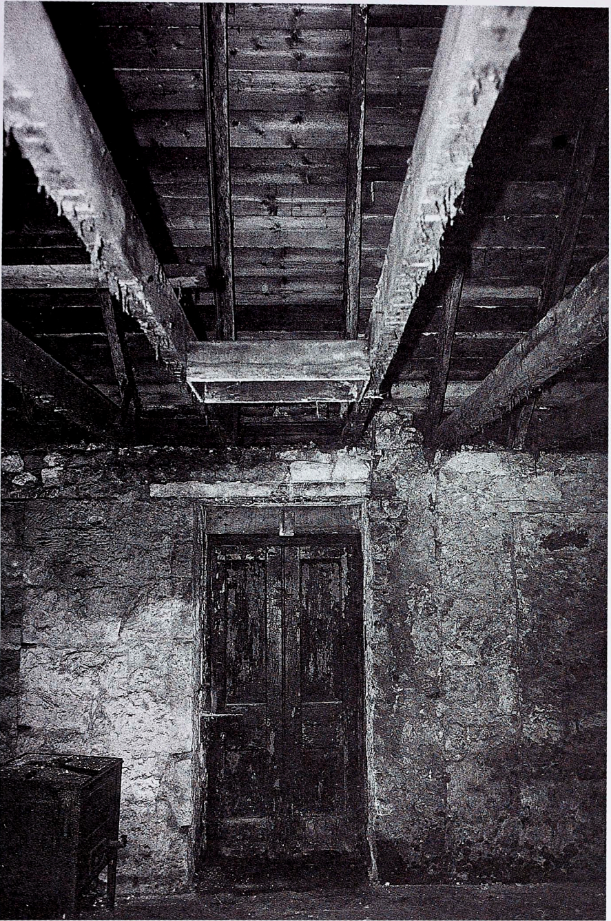
Figure 8 Interior of No. 11, west wall and door, with (to the right) evidence of gable material between the rafters, and vertical line suggesting some sort of change in the west wall.
