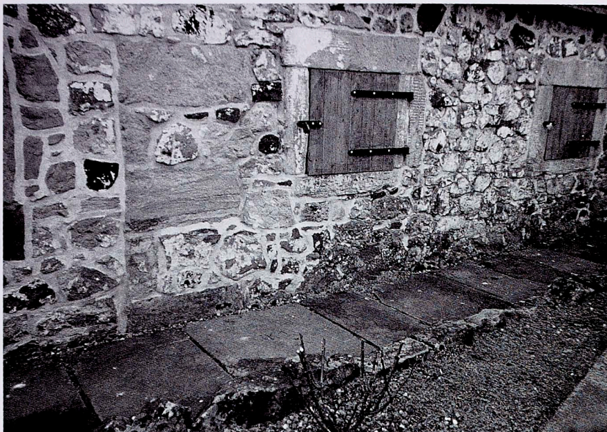
Figure 9 Back (east) wall of No. 11, showing rectangular corner stones.
