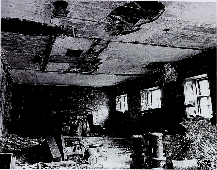
Figure 15 Interior pre-restoration, looking north; note ceiling scars delineating the lobby and room arrangement after the enlargement of the building.
