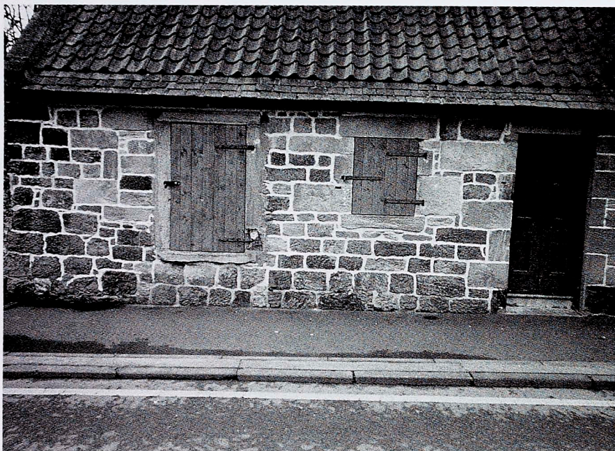
Figure 20 West wall of No. 11, showing evidence at side of larger window of a small blocked-up window which matches the small window to the right.
