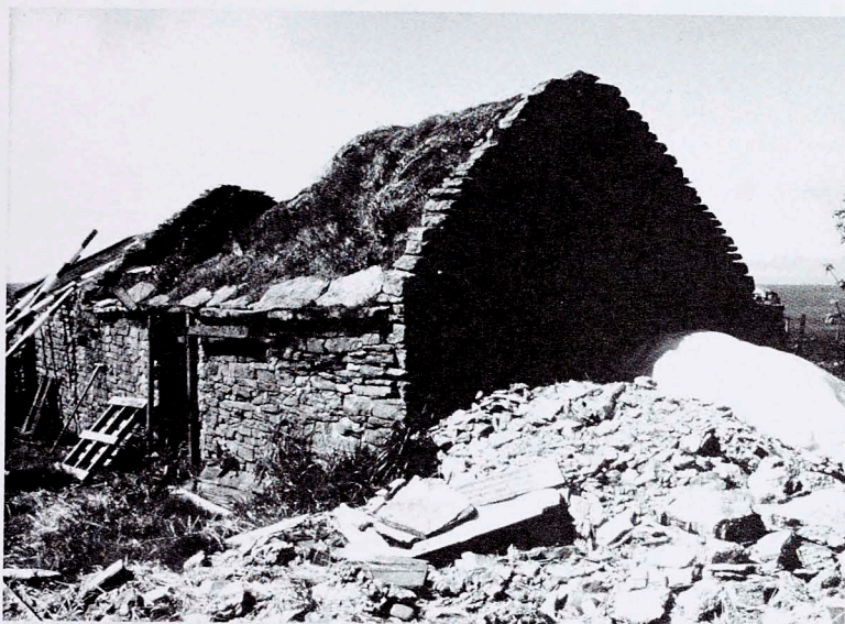
Thatched roof with curved skews and divot base layer at Greens in Toab.
