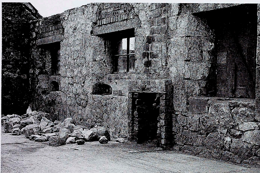
Figure 13 Interior of No. 11, showing sills of east-facing windows now cleared of loose material, revealing original stepped sills with niches.
