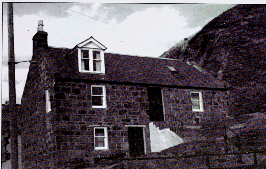
Figure 4. Crovie: Dwelling built against the slope with a two-bay cellar/fishing-gear store with independent access (now converted for domestic use). The regular upper-floor, three-bay frontage is approached by a forestair, and together with the attic, formed the family accommodation with a sea-facing gable window. The building probably dates from the first half of the nineteenth century; the dormer window is later.
