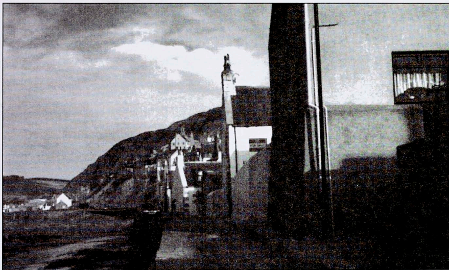
Figure 2. Gardenstown: Narrow roadway raised above the beach. Note that the houses are all gable end to the sea, facilitating greater housing density close to the shore as well as reducing the impact of gales on the dwellings. Paired gable windows facing the sea enable the occupants to watch for boats.
