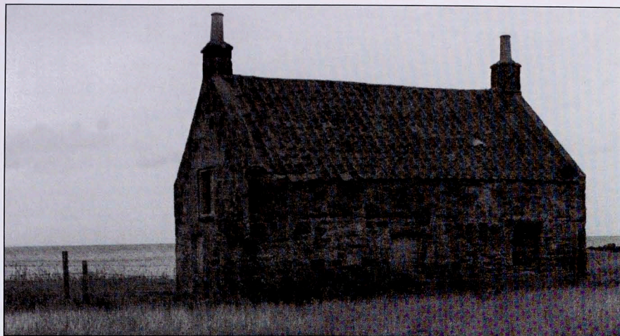
Figure 4. Rear elevation of Pitmilley salmon bothy, Fife, with the red pantiled roof and twin chimney stacks. The glass pantile is just visible. Photograph Roger Leitch, 1989.
