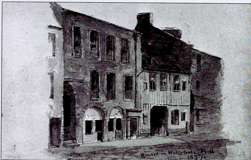
Figure 7. This is an extremely useful view of a timber-fronted building in Watergate, Perth. The last of the timber-fronted buildings in Perth, Kinnoull Lodging, was demolished in 1966. Again Lessels includes such interesting details as the shutters and the pend with canted shoulders, presumably leading to a yard at the rear. The building to the left is notable for its arched shopfront openings, still to be seen at Gladstone's Land, Edinburgh, and in Elgin, Moray. (Crown Copyright: RCAHMS SC928563)
