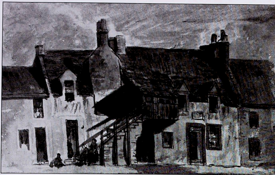
Figure 6. A view of houses in Fisherrow, Musselburgh, East Lothian, c. 1860, including, on the right, the premises of Robert Tait, a cattle dealer. The other buildings shown are presumably fisher housing. This depiction is particularly interesting for the detail of the cantilevered timber section and the timber handrail on the forestair. (Crown Copyright: RCAHMS SC928542)
