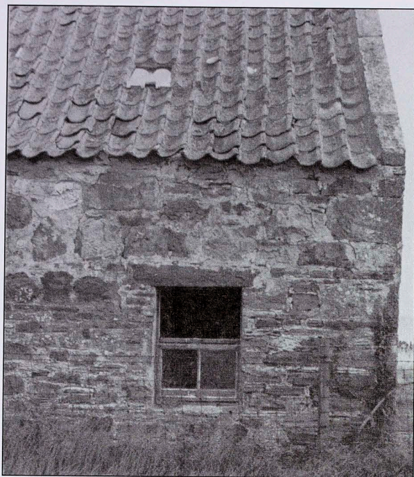
Figure 5. Close up of Pitmilley salmon bothy roof and building stone, with the glass pantile visible. Photograph Roger Leitch, 1989.
