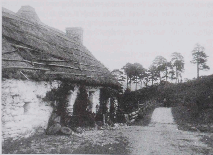
Fig. 3. Moirlanich longhouse c1900. Note the hump-back bridge crossing the burn (compare with fig. 1) and the thatched roof. The thatch is held in place by horizontal timber spars fastened to the turf underlay by hazel pins. The porch has not yet been added. (National Trust for Scotland)
