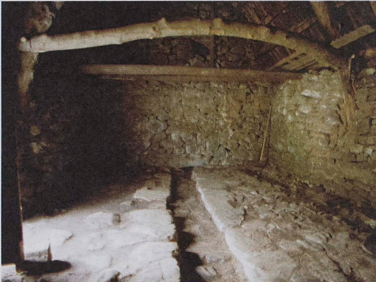
Fig. 11. The byre. Cattle would have been tethered at each side, their urine carried away by the central drain running through the gable wall.
