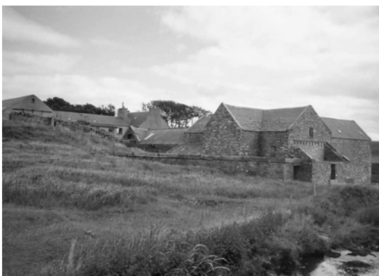
Figure 7. Kirbister Mill, Chinegar, Orphir. The most complex of Orkney's mills, Kirbister combines a grinding mill, threshing mill and kiln all on one site. Both water wheels are enclosed, and the lade allows water to be diverted to either threshing or grinding mills as required.
