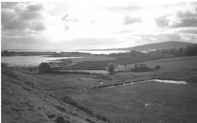
Figure 8. Firth Meal Mill. The general landscape around Firth Meal Mill showing the mill pond, mill dam, lade, bypass burn, mill cottages with threshing barn and, in the background, the L-plan three-storey mill building.
