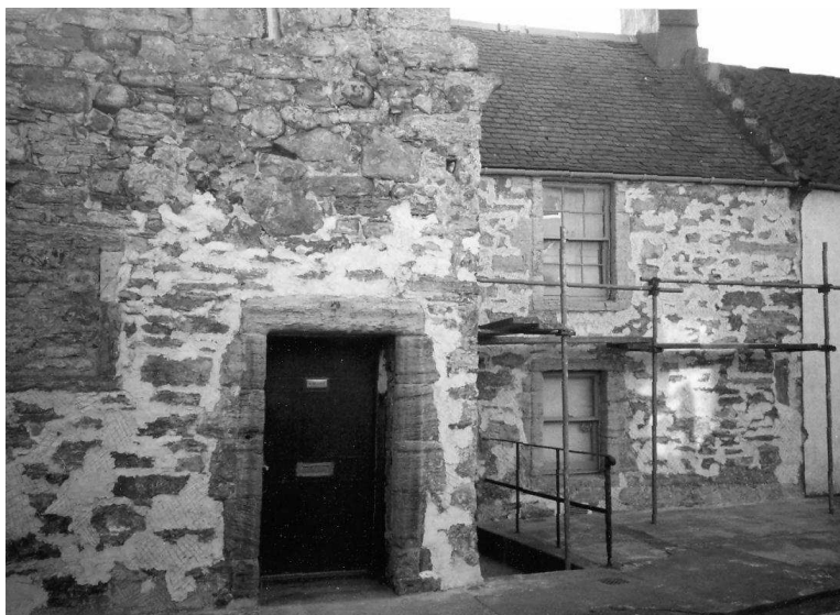
Figures 15. Dubbing and pointing: right side.
