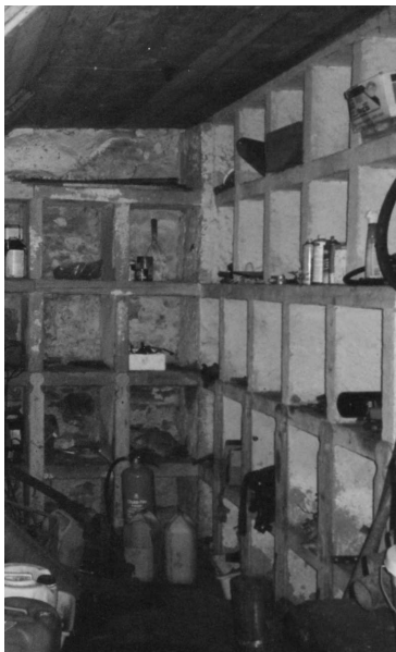
Figure 4. Many winter recesses in an outbuilding now used for general storage at Burnturk Farm, Kingskettle, Fife (IBRA Register No.1248). (Photo: P Walker, 2004)
