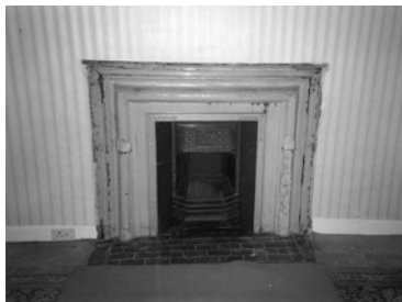
Figure 8. The first-floor chimneypiece, stripped down but unrestored.
