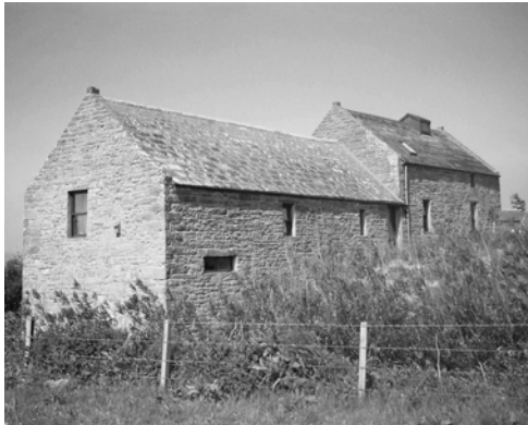
Figure 4. Kirkhouse Mill, South Ronaldsay. The horizontal slot in the wall suggests an internal wheel. Given the remoteness of the site, it is unlikely that this was to reduce noise. The wheel was enclosed more probably because of the site's exposed position – to protect it from windage, to prevent water being blown from the bucket, or to guard against ice damage.
