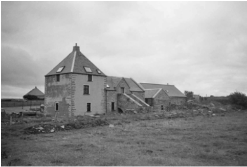
Figure 4. Kirkhouse Mill, South Ronaldsay. The horizontal slot in the wall suggests an internal wheel. Given the remoteness of the site, it is unlikely that this was to reduce noise. The wheel was enclosed more probably because of the site's exposed position – to protect it from windage, to prevent water being blown from the bucket, or to guard against ice damage.
