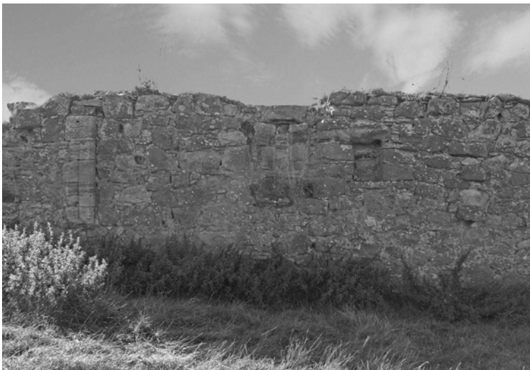
Figure 3. Blocked window, cupboard and jamb of seventeenth-century structure.
