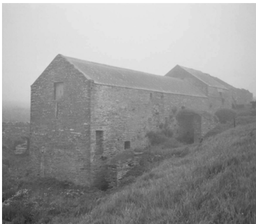
Figure 7. Kirbister Mill, Chinegar, Orphir. The most complex of Orkney's mills, Kirbister combines a grinding mill, threshing mill and kiln all on one site. Both water wheels are enclosed, and the lade allows water to be diverted to either threshing or grinding mills as required.
