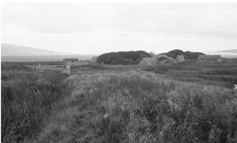
Figure 14. Kirbuster Mill, Birsay. The earthworks upstream of the mill suggest that the lade was not carried on stone piers, as was the case in the later mills, but took the form of a specially cut watercourse travelling in a straight line from the substantial dam to the mill. The bypass burn can be seen on the right side of the picture, and the farmstead associated with the mill is visible in the background.
