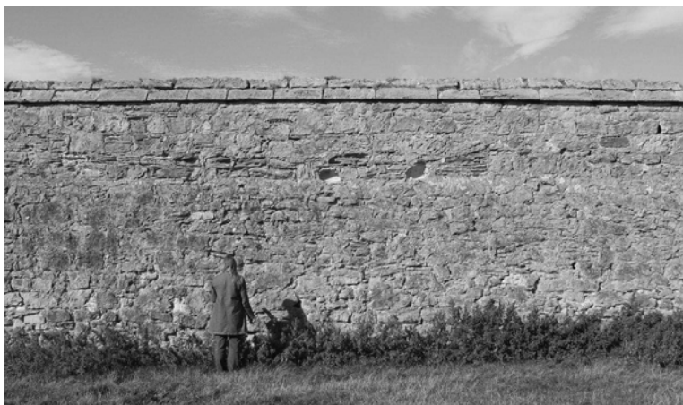
Figure 4. The walled garden: note the raising of the wall, and the pitched copes.
