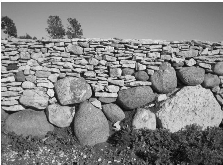
Figure 4. The contrast between granite fieldstones and limestone is dramatically revealed in this section of repaired wall by Kaja Juulik.
