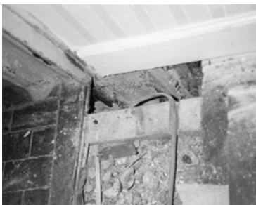
Figure 9. Detail of the first-floor room, showing part of a stone chimneypiece and wallpaper beneath floor level.
