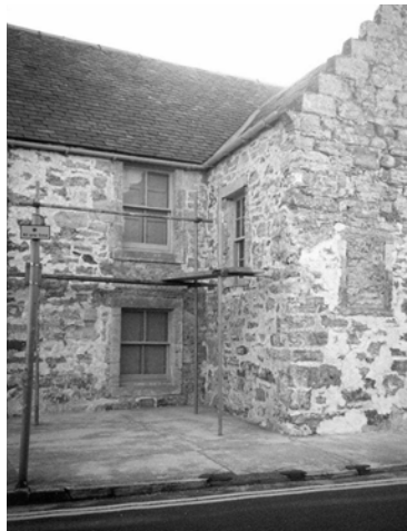
Figure 14. Dubbing and pointing: left side.
