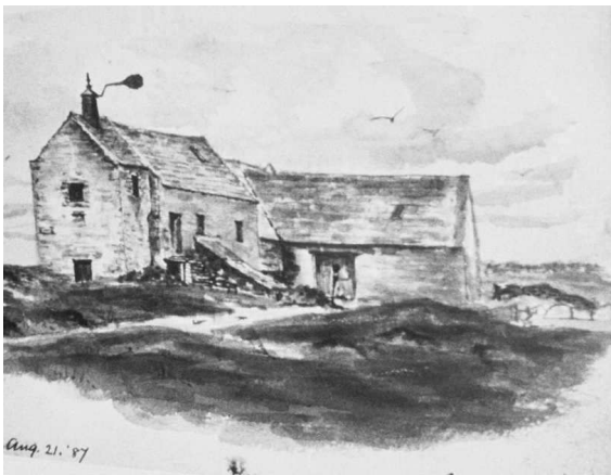
Figure 6. Mill of Cairston, Stromness. This appears to have featured both an overshot and an undershot wheel placed in sequence. A take-off from the dam leads the water to the overshot wheel and the runoff from here runs into the sump for the undershot wheel. The main evidence for two wheels comes from the two square shaft holes.
