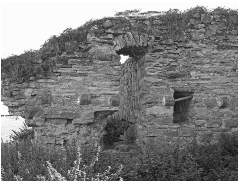
Figure 1. Doorway in the south wall of the 'castle', with the corbels clearly 'cutting through' the opening.
