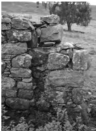
Figure 3. One of the cruck-slots is visible just east of the doorway on the south side of the kilnbarn at Sliabhclachd, NJ02SE 29. (RCAHMS, DP 019125; Crown Copyright: RCAHMS)
