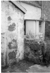
Figures 20 and 21. Partition wall and collapsed wall of outhouse.
