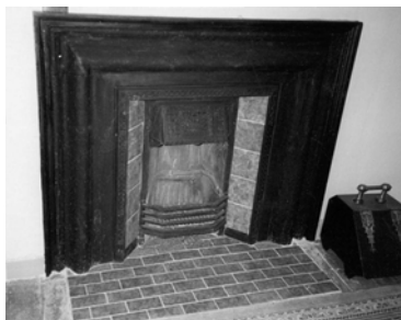
Figure 10. The first-floor chimney-piece after restoration.
