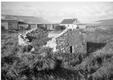
Figure 12. Kirbuster Mill, Birsay. Upstream wall and gable, the latter showing the aperture for the shaft.
