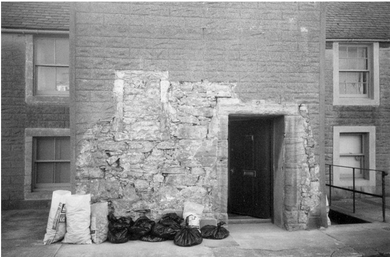
Figure 11. Removing the cladding, 2006.
