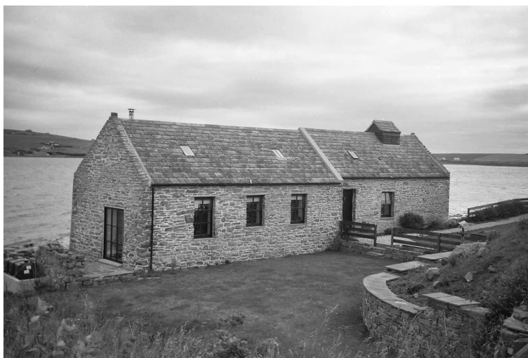
Figure 11. Cara Corn Mill, South Ronaldsay. Cara is a small, linear corn mill which originally featured a breastshot wheel (now absent). The kiln block, to the right, is a later addition to the original building.
