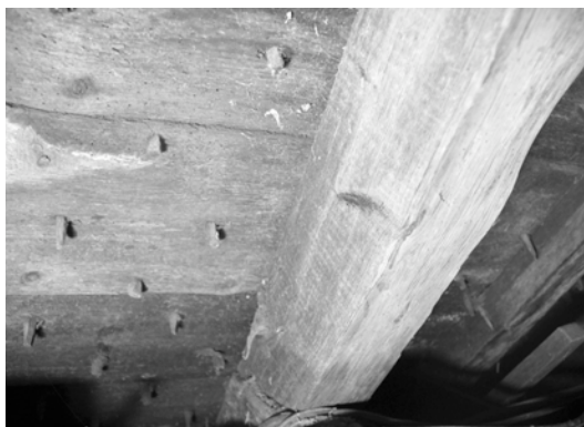
Figure 4. Sawn and hewn pine baulks in the roof of the Old Courthouse, Campbeltown. Note the wooden pegs in the sarking.
