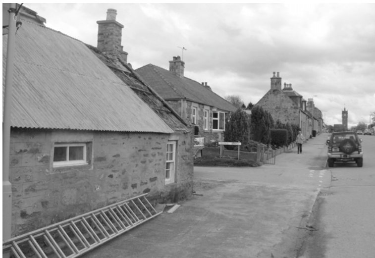
Figure 4. The former smiddy building from the west, at the moment when the tin roof was removed and the thatch roof exposed for the first time in decades. Also visible is the curiously small window in the front wall, which appears to have been formed by blocking up a larger opening.
