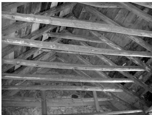
Figure 7. Small, fast-grown hewn pine timbers in the roof over the Old Laundry, Drum Castle (c.1800).
