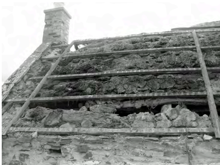
Figure 6. The rear roof shows few remnants of the straw thatch finish, although the turf divots are clearer to view. The partial collapse of the sarking battens and their sods provides glimpses of the varying thicknesses of sarking. Also recorded here are the later brick chimneyhead and the rather fine stone skews.
