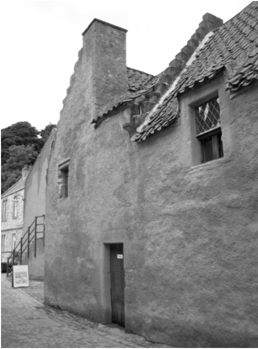
Figure 7. Culross Palace, Fife (1597–1611) – mural chimney and crow-stepped gable.
