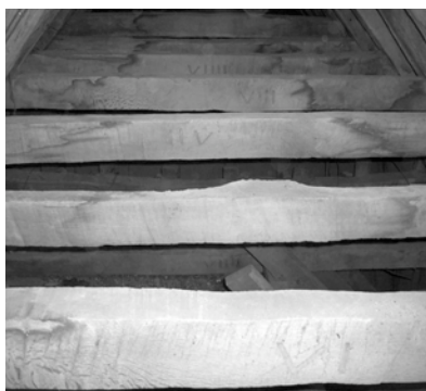
Figure 5. Hand-sawn oak collars in the roof of the Mansion House, Drum Castle.
