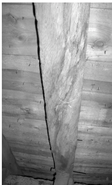
Figures 3a and 3b. Bastard-grained oak timbers in the roof of the Mansion House, Drum Castle.
