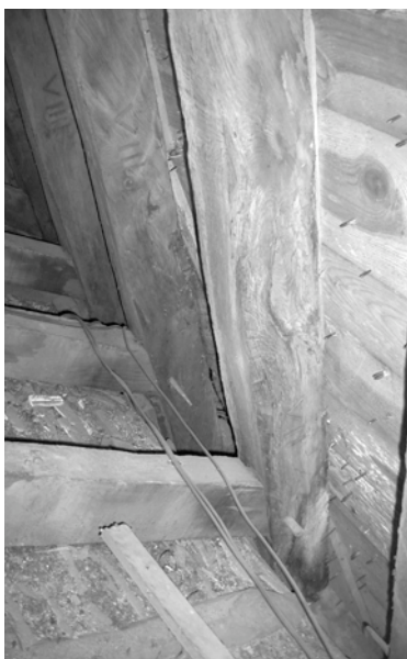
Figures 3a and 3b. Bastard-grained oak timbers in the roof of the Mansion House, Drum Castle.
