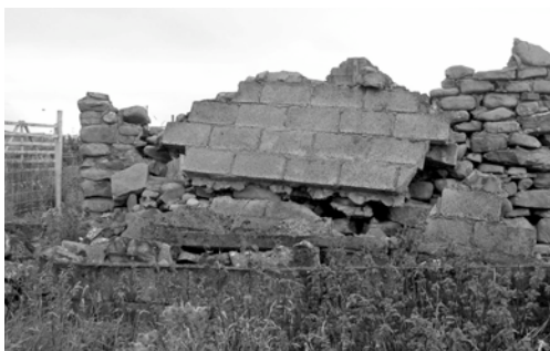
Figure 13. A collapsed gable showing the damage from rebuilding the walls of the shells of the old houses with concrete blockwork as part of a filmset in the early 1980s.
