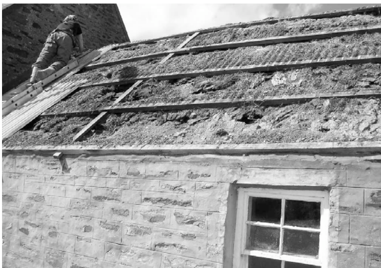
Figure 5. The tin roof in the course of removal. The previous straw thatch finish is visible, although now pressed down into a corrugated pattern. The turf divots below are most clearly seen between the tin roof battens along the lower section of roof. The substantial front stone wall has been extensively pointed using a cement-based mortar and then lined out. Note the slightly unusual 8-pane sash-and-case arrangement of the eastern window.
