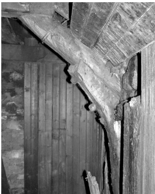
Figure 9. Detail of the pegged joint between the cruck blade and stub post (crup).
