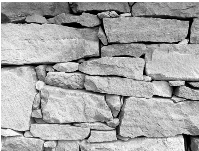
Figure 5. Finely executed masonry to the front wall of the house, shaped from Torridonian sandstone.
