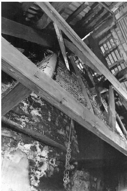
Figure 6. Camserney Longhouse, Perthshire (mid-18th century): hanging chimney. (© Crown Copyright: RCAHMS. Licensor www.rcahms.gov.uk)
