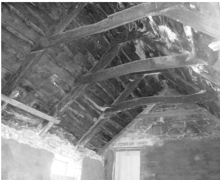
Figure 7. Interior view looking south-west (after clearing out and the creation of a new door opening to link to main house). The substantial main roof trusses at wide centres are constructed using irregular timbers, which is most clearly seen in the lack of straightness in some of the tie beams. Several of the trusses have small tie beams near their apex, and all are beam-filled at their wallhead ends. The irregular sarking battens are clearly visible, as well as the base of earth and clay material which was applied from above between their spacings.
