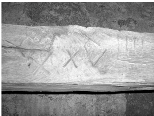
Figure 2. Duplicate carpenters' marks on oak in the roof of the Mansion House, Drum Castle.
