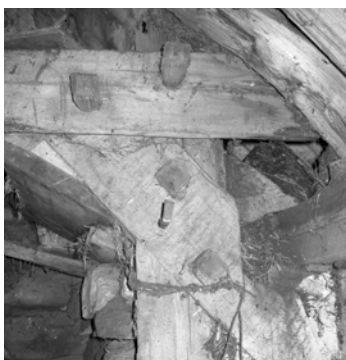
Figure 6. Hand-sawn pine in a composite cruck in the Inverey byre.
